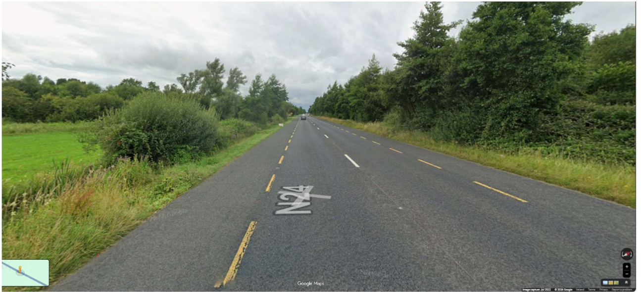
Figure 2 – Existing N24 on section proposed for Grid Connection (Source Google Street view (July 2022))
